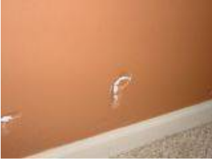
Photo 15 Drywall Damage
